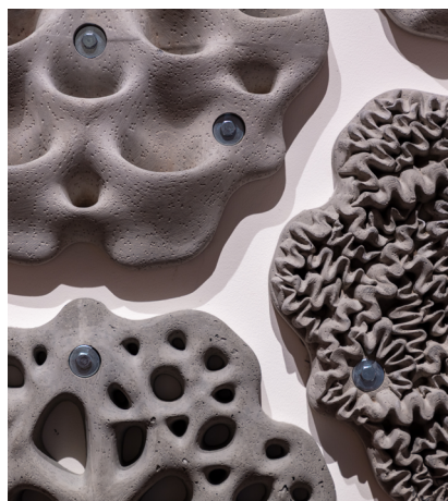
DETAIL AND INSTALL SHOTS: LIVING SEAWALL PANELS (2018), REEF DESIGN LAB, SYDNEY INSTITUTE OF MARINE SCIENCE. LOW CARBON CONCRETE, COMPOSITE REINFORCEMENT. COURTESY REEF DESIGN LAB, LIVING SEAWALLS AND ALEX GOAD.
